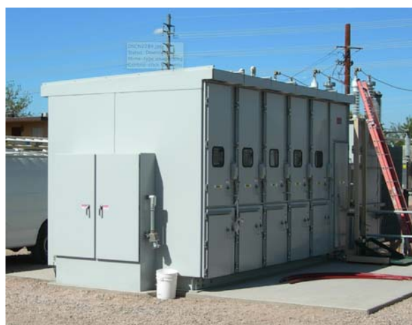
Figure 6. A small bank of medium voltage switchboxes shows both weather-tight and RF-tight enclosures. Such systems have very low spurious emissions.
